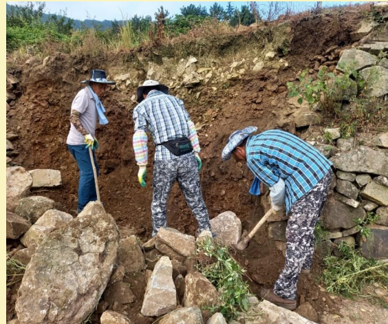
[Restoration and repair of Gudeuljang Rice paddy]
